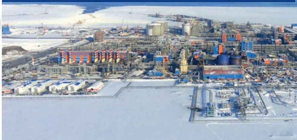
Novatek's Yamal liquefied natural gas facility on the Yamal Peninsula in the Arctic. IMAGE: NOVATEK
