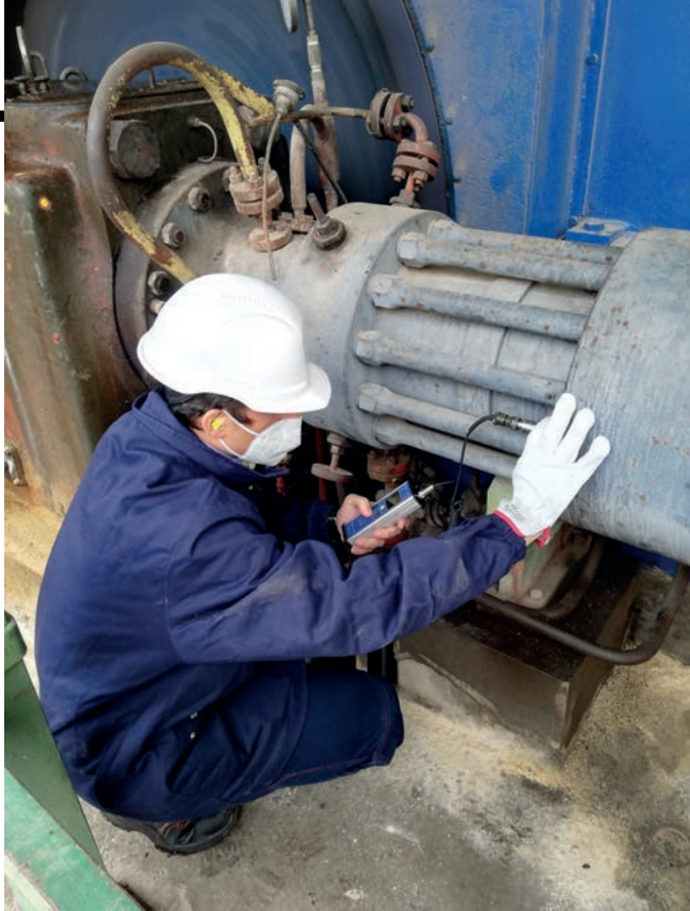
Old Esslingen hyper compressor vibration measurement. Together with LDPE case (2nd case) with the big-end rod
