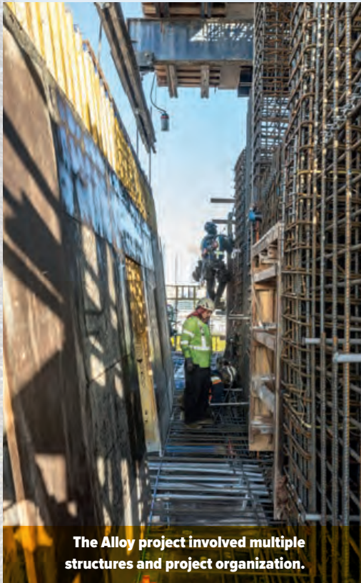
On the Alloy project, crews integrated loading platforms into the protection screen for inbound and outbound loading of equipment.
