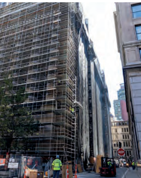
Workers watch as the Kewazo LIFTBOT moves materials to numerous floors.
