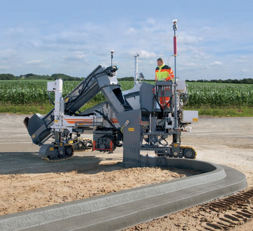
Minnich has a Control Speed Vibrator (CSV) with which contractors can choose the speed they want the vibrator to run based on the workability of the concrete
