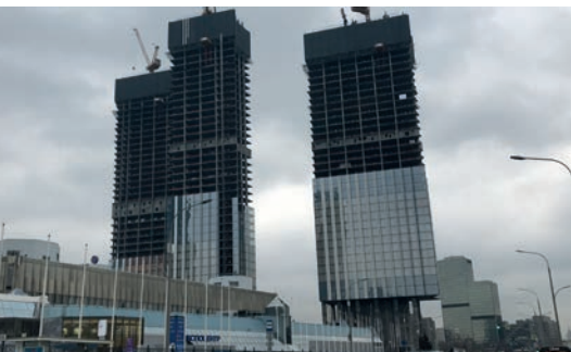
Moscow remains Russia's biggest market for construction tower cranes
