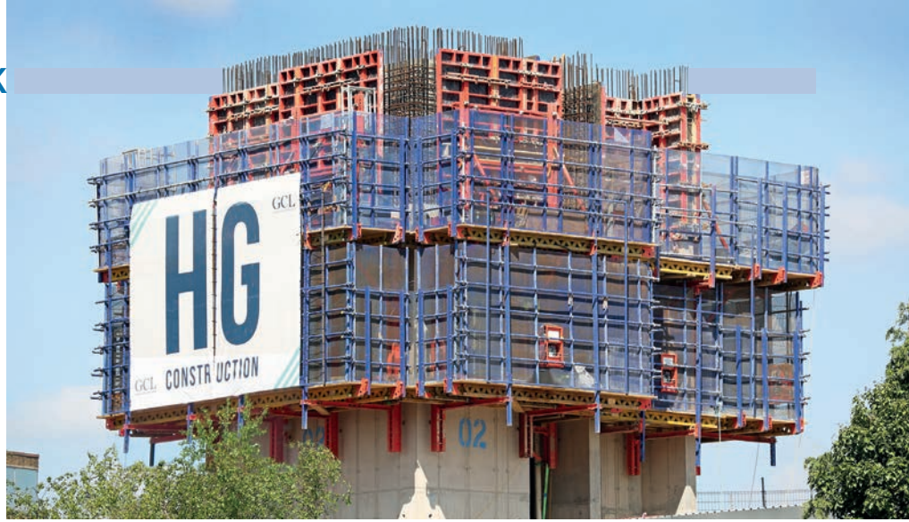
The RCS MAX Hydraulic Unit allows several platforms to climb a structure simultaneously
