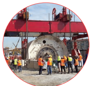
416 ton: Transport, Lowering and Installation
