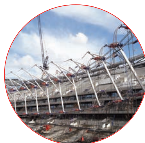
216 Strand Jacks working simultaneously
