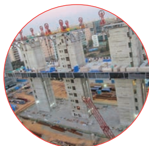
Installation of 10 complete Floor Slabs : Strand Jacks
