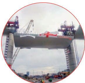
Installation of sections weighing up to 2,000 ton
