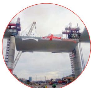
Installation of sections weighing up to 2,000 ton
