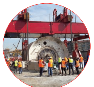
416 ton: Transport, Lowering and Installation
