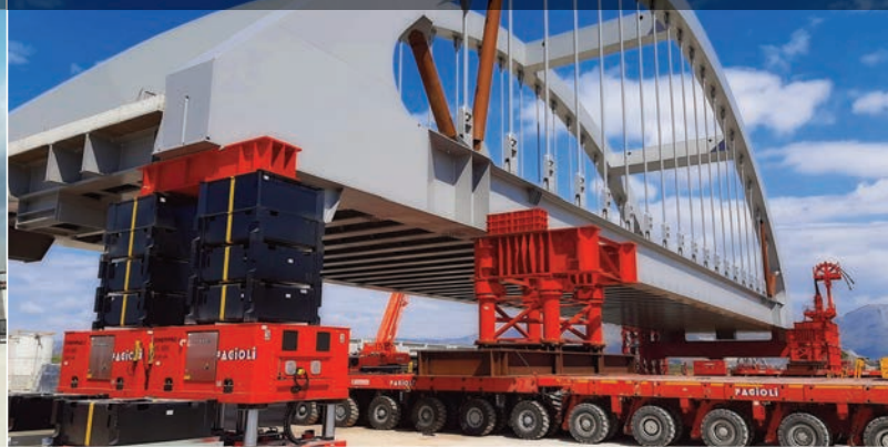
Transport, lifting and Installation of a 2,000 ton bridge in Italy by means of 500 ton jack-up system, strand jacks and SPMTs
