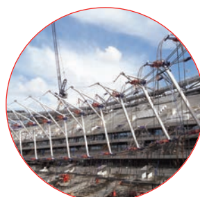
216 Strand Jacks working simultaneously
