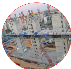
Installation of 10 complete Floor Slabs : Strand Jacks
