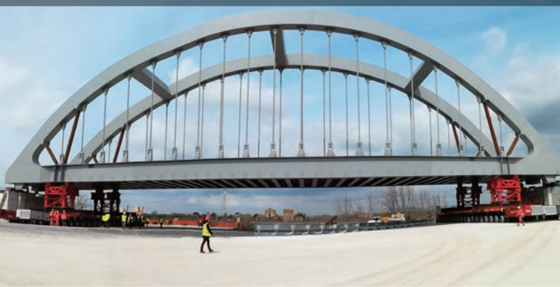
Transport, lifting and Installation of a 2,000 ton bridge in Italy by means of 500 ton jack-up system, strand jacks and SPMTs
