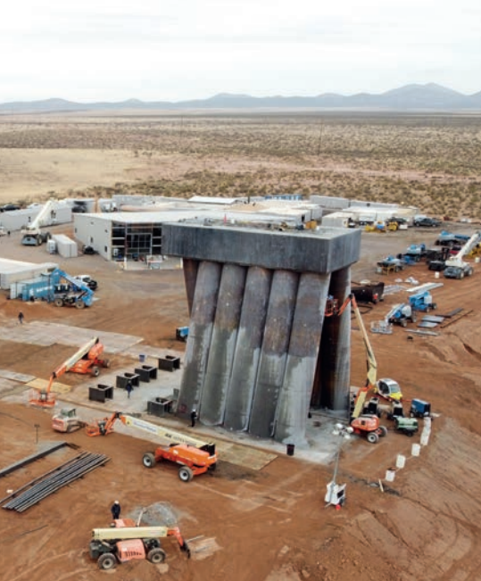
Sarens lifted a launch chamber for spaceflight technology company SpinLaunch
