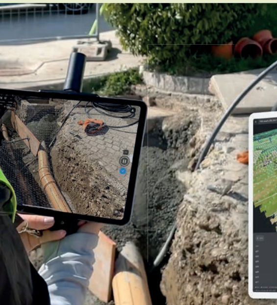
PIX4D'S MOBILE APP PIX4DCATCH USES YOUR PHONE OR TABLET CAMERA TO TAKE PHOTOS WITH THE CORRECT AMOUNT OF OVERLAP NECESSARY FOR RECONSTRUCTION
