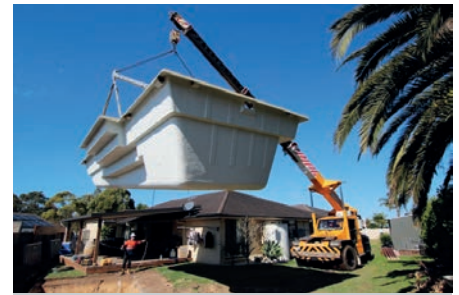
Australia-based A.J. Scarr completed a pool installation with a Terex Franna AT20
