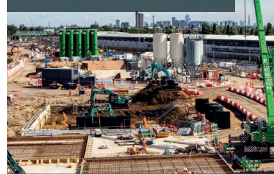
CONSTRUCTION WORK IS ONGOING ON THE LONG-RUNNING HS2 PROJECT PHOTO: HS2
