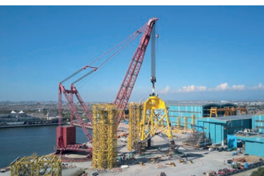
The offshore wind turbine bases consist of upper (pictured) and lower jacket sections topped by a transition piece to connect the jacket and the turbine tower
