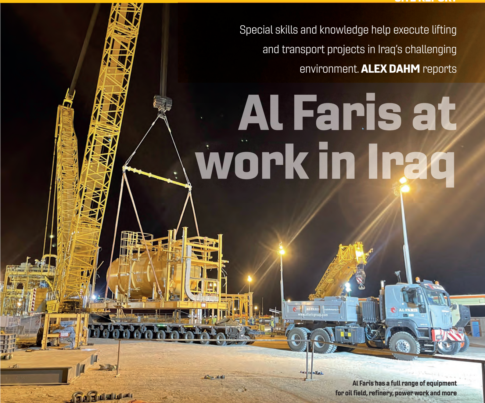
Refinery vessel installation at the WQ1 oil field
