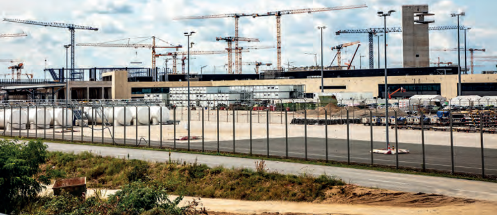
Twelve BKL cranes are being used at the airport
