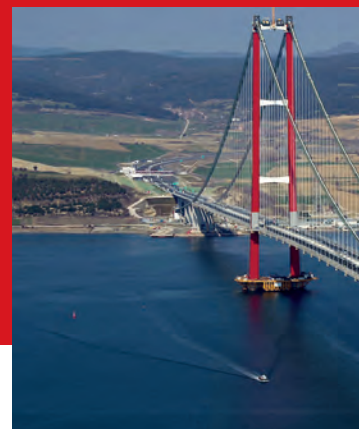
PHOTO: MARR CONTRACTING
