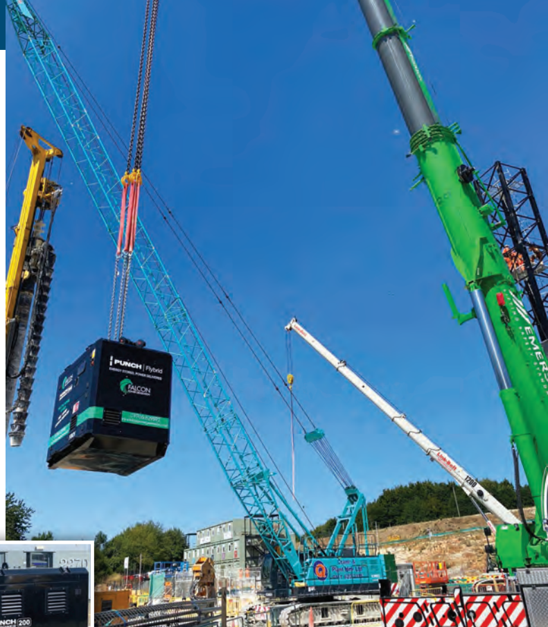
Installing a punch Flybrid energy storage unit on a HS2 railway construction site at Little Missenden in the UK
