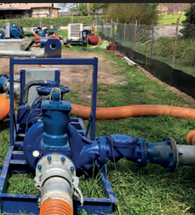
PHOTO: HOLLAND PUMP
