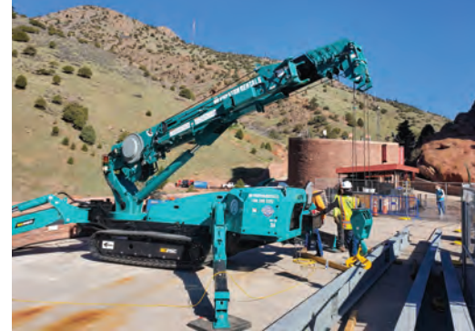
The crane was used to hoist steel beams utilizing a below-the-hook beam clamp.
