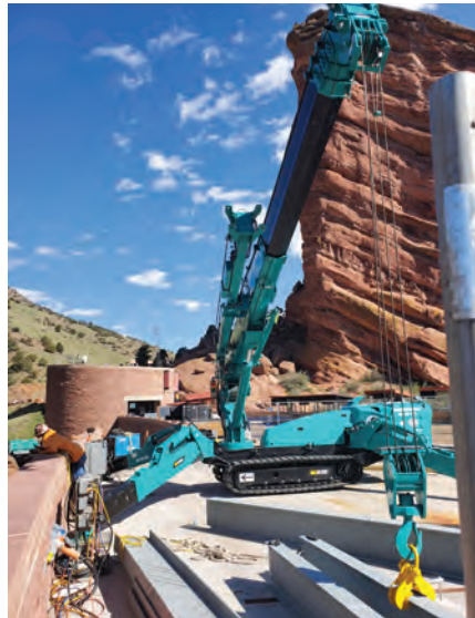
The MC815 was selected because it could travel in on the paved surface on its bolt-on rubber track pads, rapid set up and ability to hoist in a limited access area.
