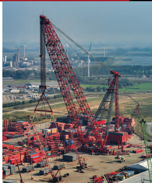
The Mammoet PTC35 lifts a steam generator at Bruce Power, Ontario, Canada.
