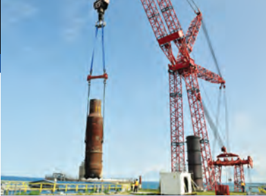
SGRT guides one of the eight new steam generators back into Bruce A with the PTC-35 crane.
