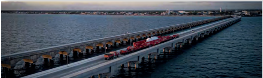
Mayan train works kept the route constantly changing, and at the Yucatan peninsula several civil works were made to navigate around the building sites, causeways and tollbooths.
