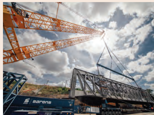
Sarens Giant Crane, Little Celeste, replaces two enormous century-old rail bridge sections in Massy, France.
