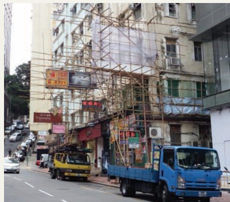
Bamboo scaffolding in Hong Kong.
