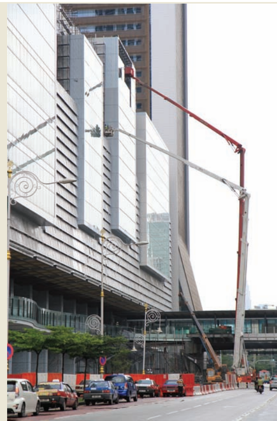
Two of Keng Guan Skylift's truck mounts fit glass facades on a building in Kuala Lumpur.
