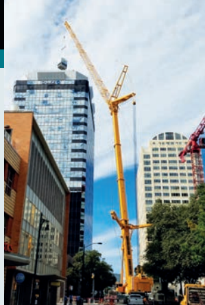
Alamo's Liebherr LTM-1500-8.1 performed the 300-foot lift at a 235-foot radius.
