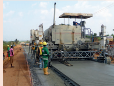
Wirtgen's SP 500 slipform paver at work in Nigeria
