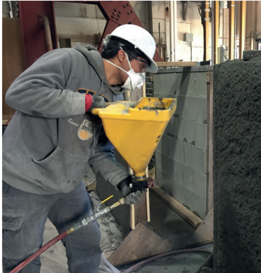
Plastering a wall with earthquake-resistant concrete
