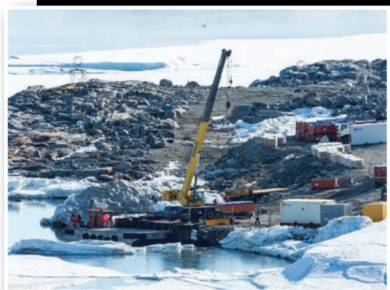
The Grove RT540E rough-terrain crane working at the Australian Antarctic station
