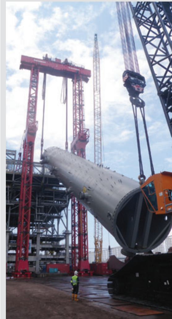
The absorber was lifted using a 'top and tail' operation
