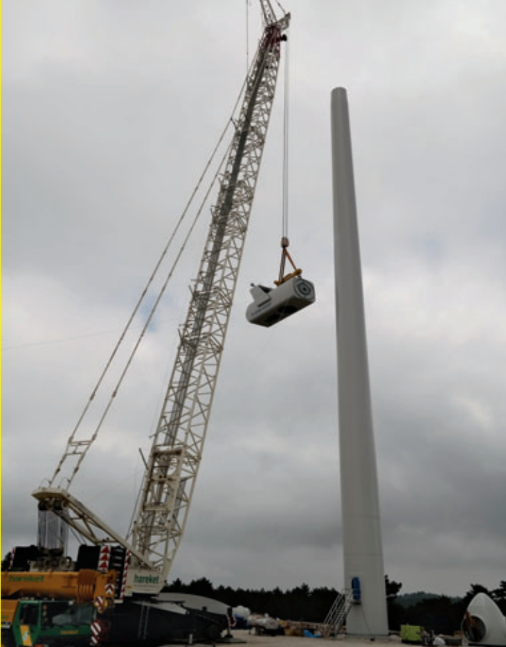
Transportation and installation of 5 units Vestas V100 turbines at Balikesir Turkey.
