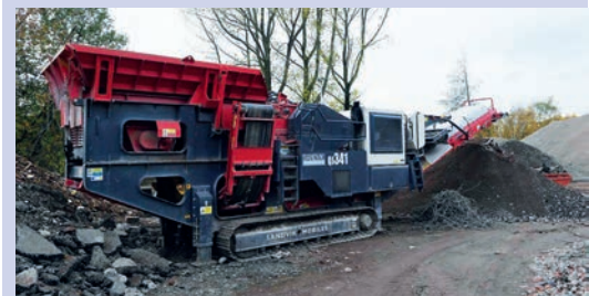
A Sandvik QJ341 on site for SJ Walchester
