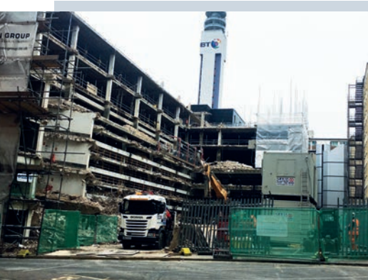
Garic welfare facilities at the Coleman site
