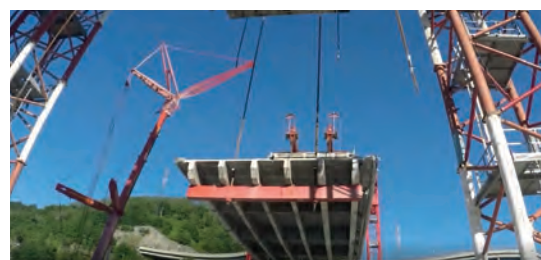
Dismantling the western piles (top) and the removal of beam 11 of the Morandi Bridge in a secure operation
