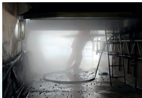
Aquaforce carries out high pressure water jetting under the Ouse bridge
