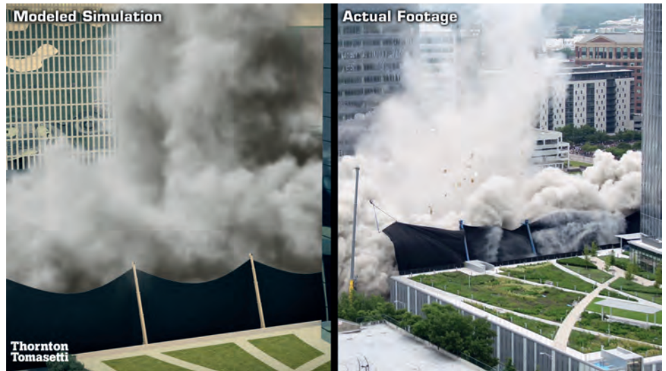
Thornton Tomasetti's structural engineers also developed plans for the mechanical demolition of the below-grade car park and determined the structural stability of the building prior to the implosion...
