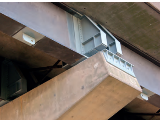
New jacking points in place on the bridge
