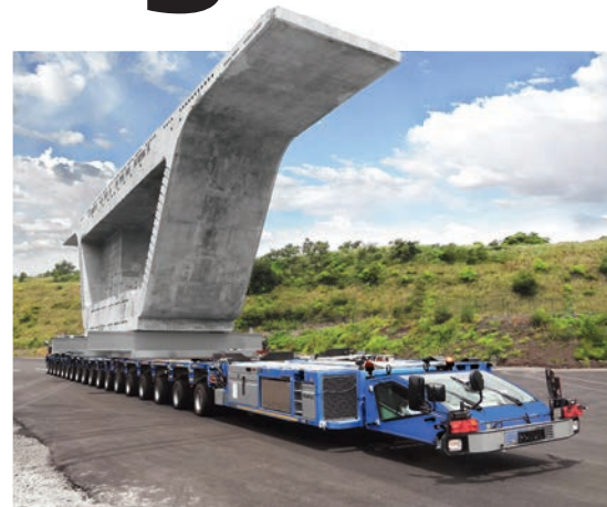
A Goldhofer PST/SL being used to transport a bridge section for contractor Vinci on La Réunion island
