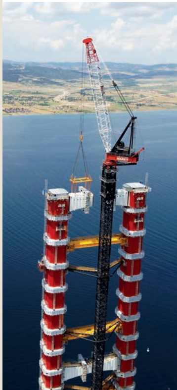
The 155 tonne section of the UCB (upper cross beam) being lifting into position onto the bridge towers 318 metres above sea level
