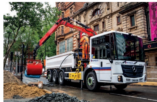
The Epsilon crane on this new Mercedes Econic for Eurovia Contracting in the UK lifts 3.7 tonnes and has an outreach of 8.2 metres
