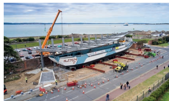
Allelys skidding the landing craft into position
