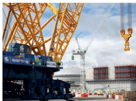
The SGC-250 will lift prefabricated nuclear reactor parts out of the domed building and slew them into position
