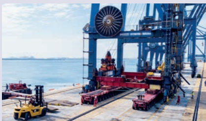
The biggest STS crane the SPMT moved weighed 1,365 tonnes
