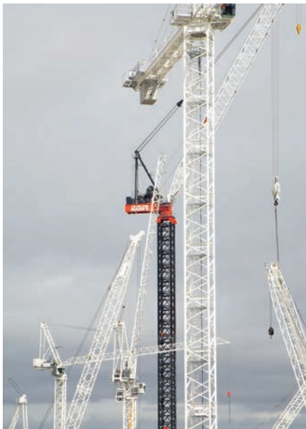
The M2480D was erected on 72 metres of freestanding tower
