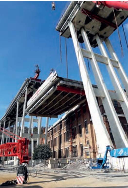
Close proximity to surrounding buildings was one of many challenges
