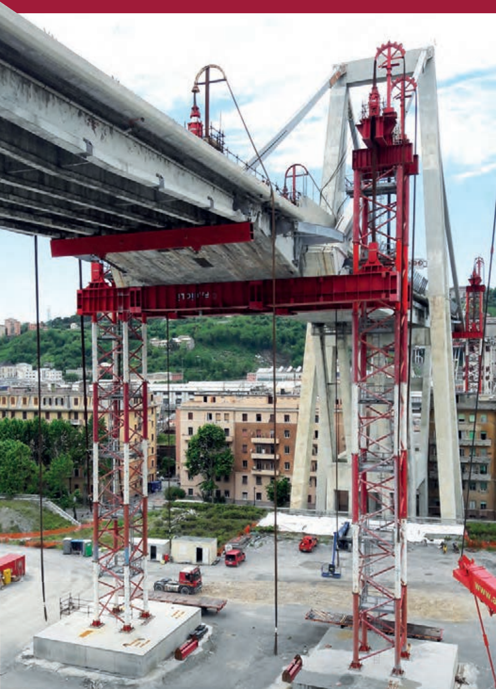
Fagioli prepares to lower the first piece in the demolition of the Ponte Morandi in Genoa, Italy
