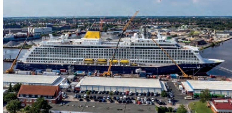
Two LTM 1250-5.1s and a Liebherr LTM 1100-5.2 were used by Ulferts
