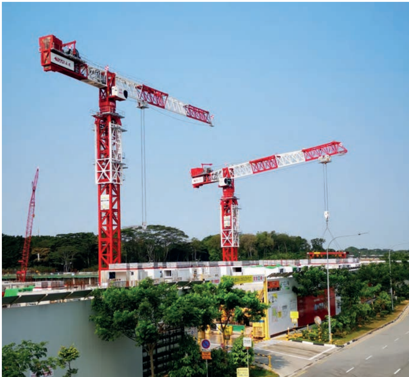
Yongmao STT1330 Max lifting 64ton in Singapore
