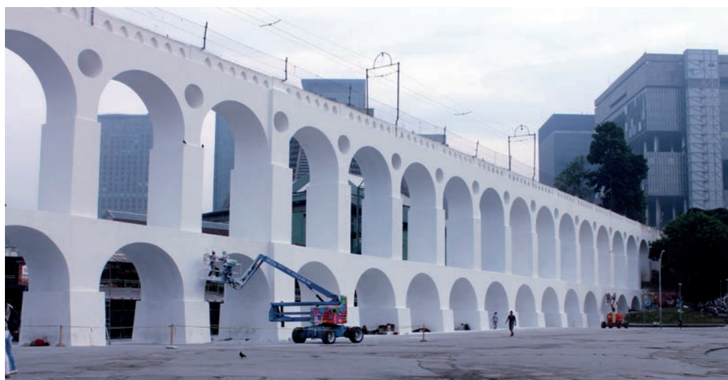
The Carioca Aqueduct is an aqueduct in the city of Rio de Janeiro, Brazil.
