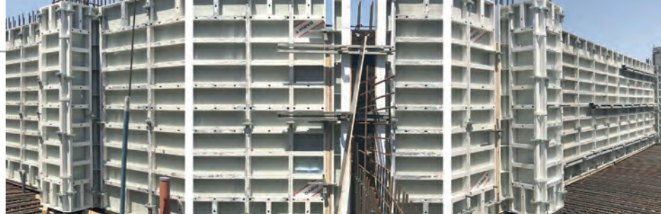
Meva's AluFlex formwork was used to construct a new building at The English College in Dubai
