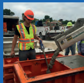
One of Betonblock's moulds being filled with concrete
