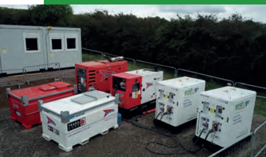
Two diesel generators were each linked to a Gridtogo energy storage unit
