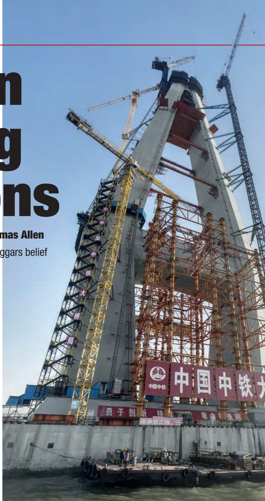
One of the record-breaking 325m-tall pylons of the Shanghai-Nantong Yangtze River Bridge
