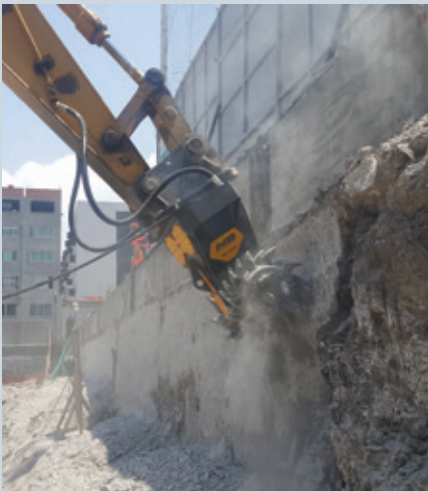
The MB-R800 is one of three models in the range and works with excavators from 10 to 22 t
