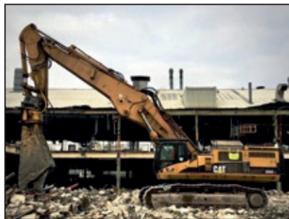
CAT 385 C fitted with a shear attachment
