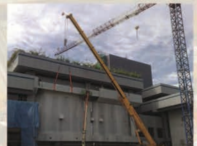
Singapore Changi Airport Terminal 1
