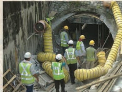
Structural Strengthening to Box Culvert Across PIE
