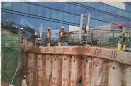
Contract 855 Circle Line Project
