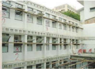
Internal Structure Demolition For New Construction. NUS, Bukit Timah Campus
