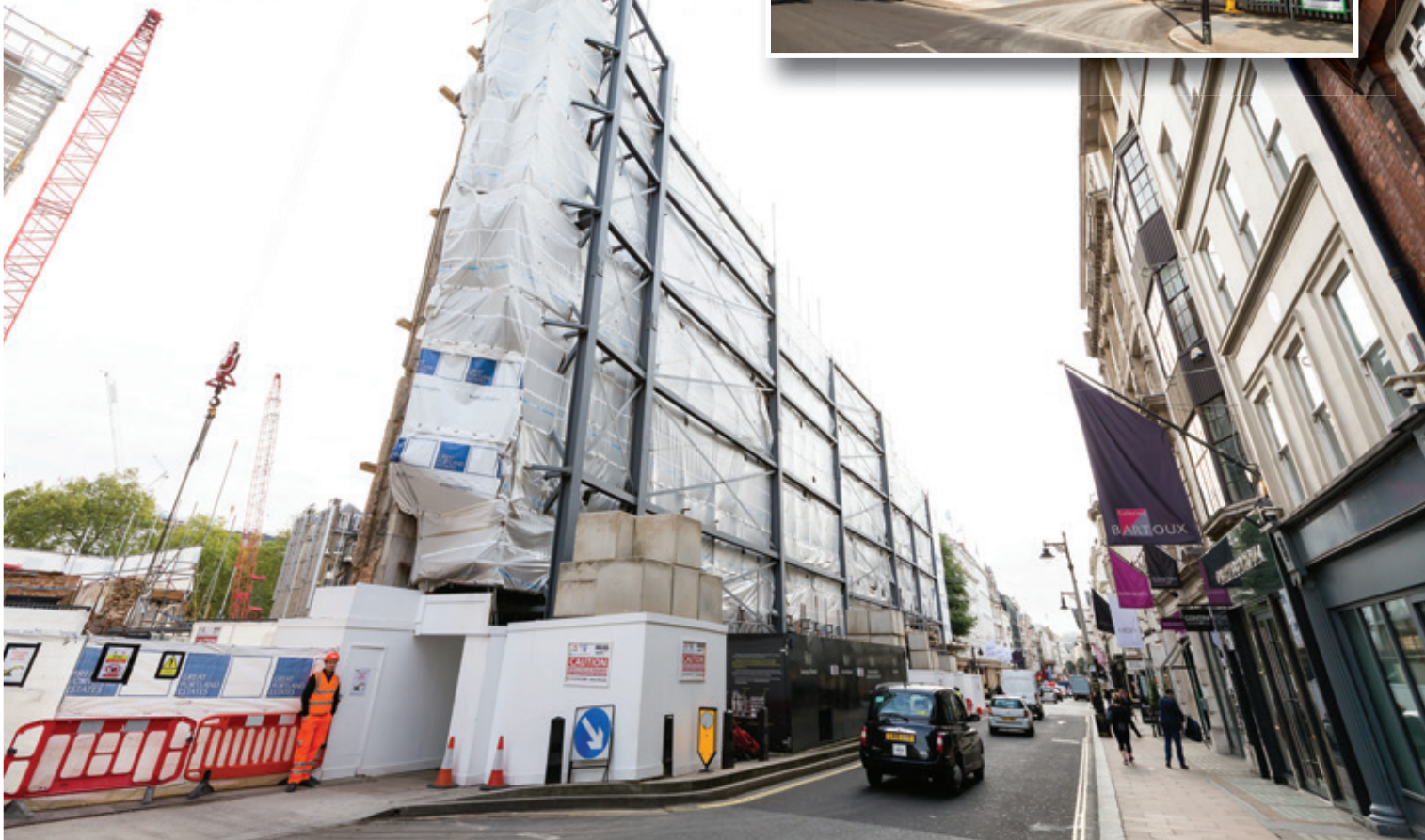
Hanover Square: 'A lot of work in London is about façade retention'
