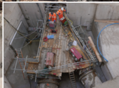
above: GNAT UK's robotic demolition team utilising a specially adapted Mast Climber to deconstruct the reinforced concrete structure during a recent top-down demolition project
