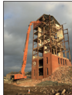
40m on hire to Caskie Demolition Scotland
